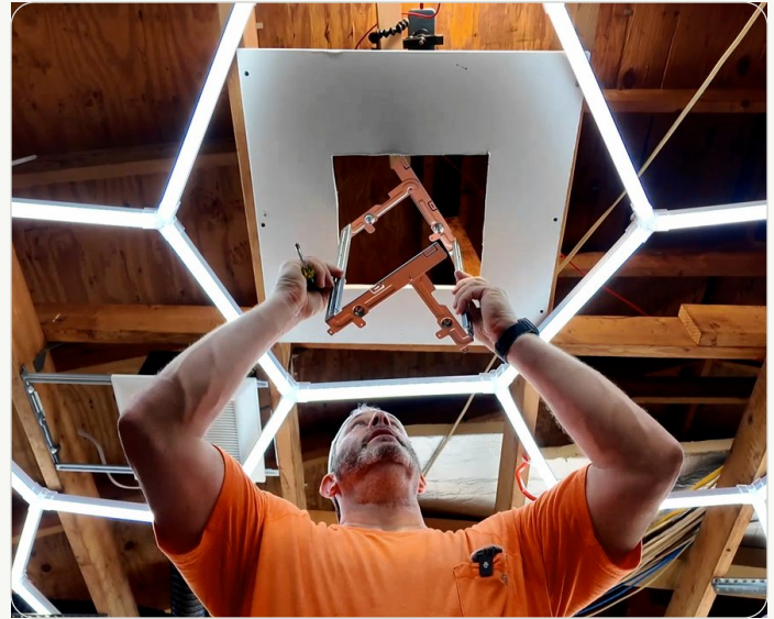
2 FOLD THE BRACKET TO PASS IT THROUGH THE OPENING
