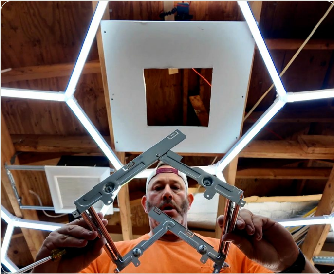
1 PRE-START THE FOUR FRAMING SCREWS
